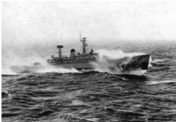
Figure 2- A frigate slamming in rough weather, from Lloyd (1989).
