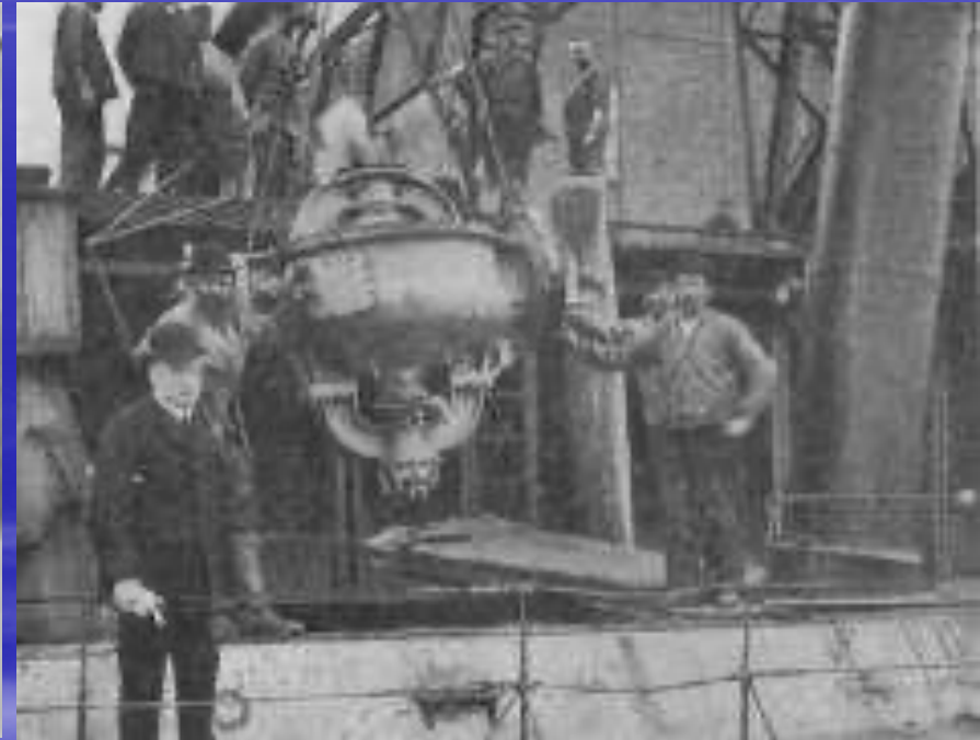
Gyrostabilizer experiments being carried on the "Sea-bar" torpedo-boat
